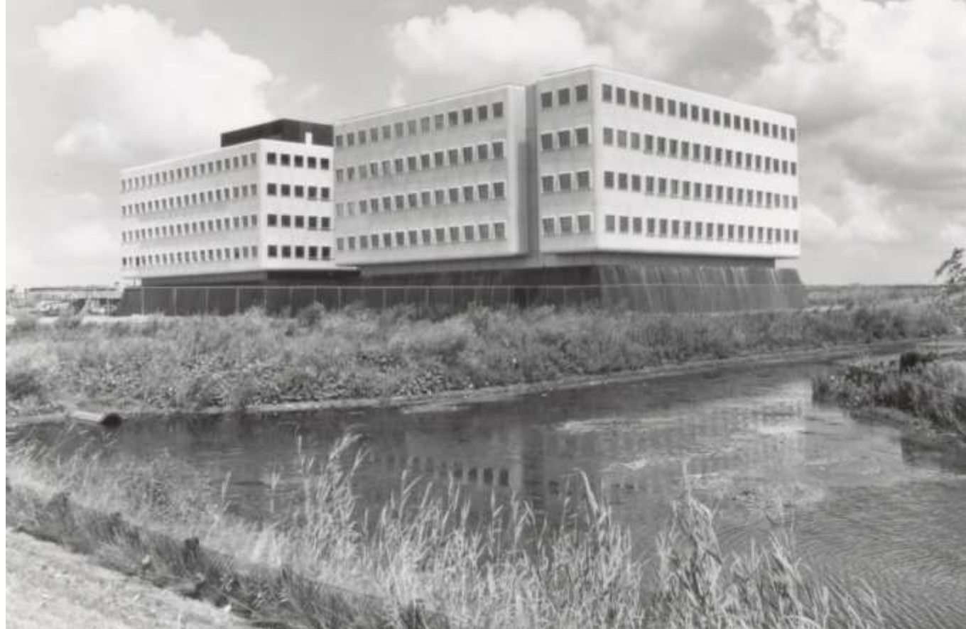
Computer Uitwijk Centrum 1982 Architect F. Balm
