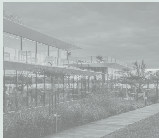
Mist Restaurant Pavillion
